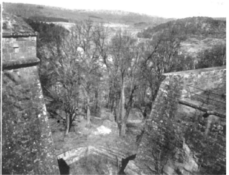
Above, the camera looks northeast from the parapets of the Citadel of Bitche. Left, an aerial view of the Citadel and surrounding terrain. We waited three months for the climb to the top.
