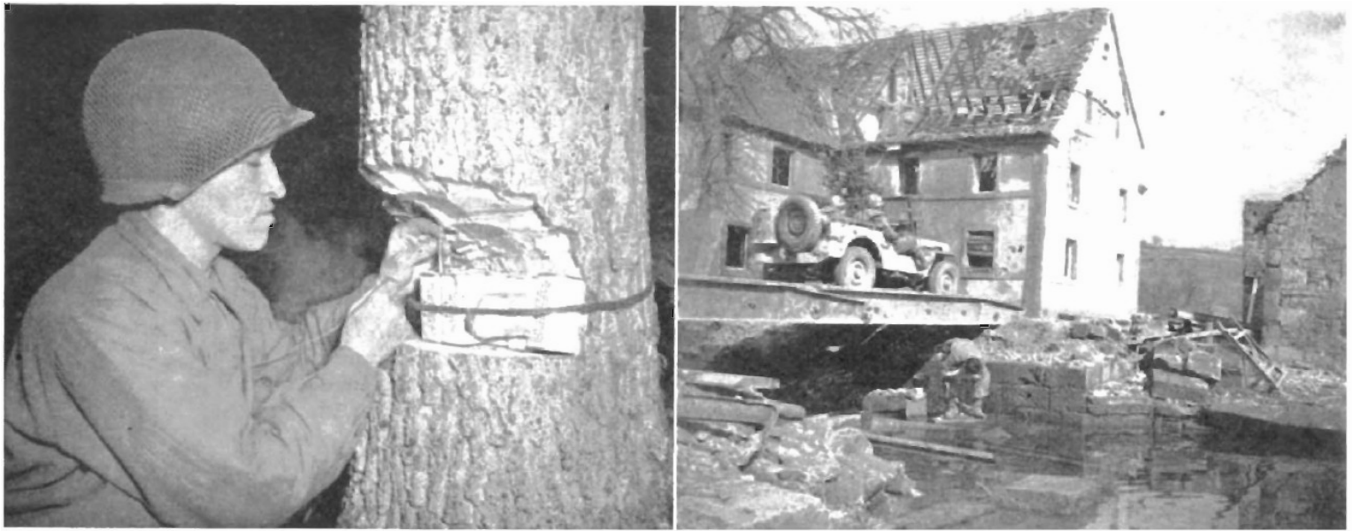
Left, tying dynamite into a notched tree. When the charge is exploded, the tree falls across the road forming an abatis, or roadblock. Above, time out to wash up.
